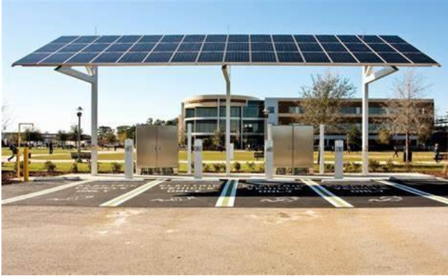
Fig. 2. Implementation of solar based charging station [14]
