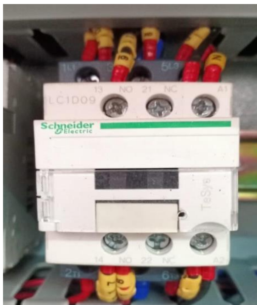
Fig. 10 Magnetic contactor
