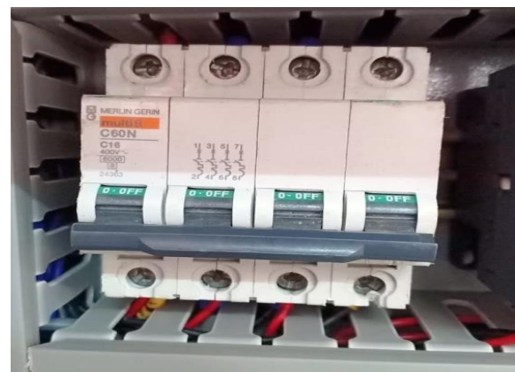
Fig. 12 Circuit Breaker
