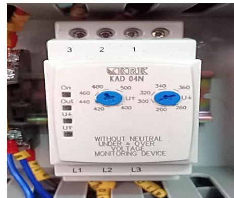
Fig. 8 Over-under voltage relay
